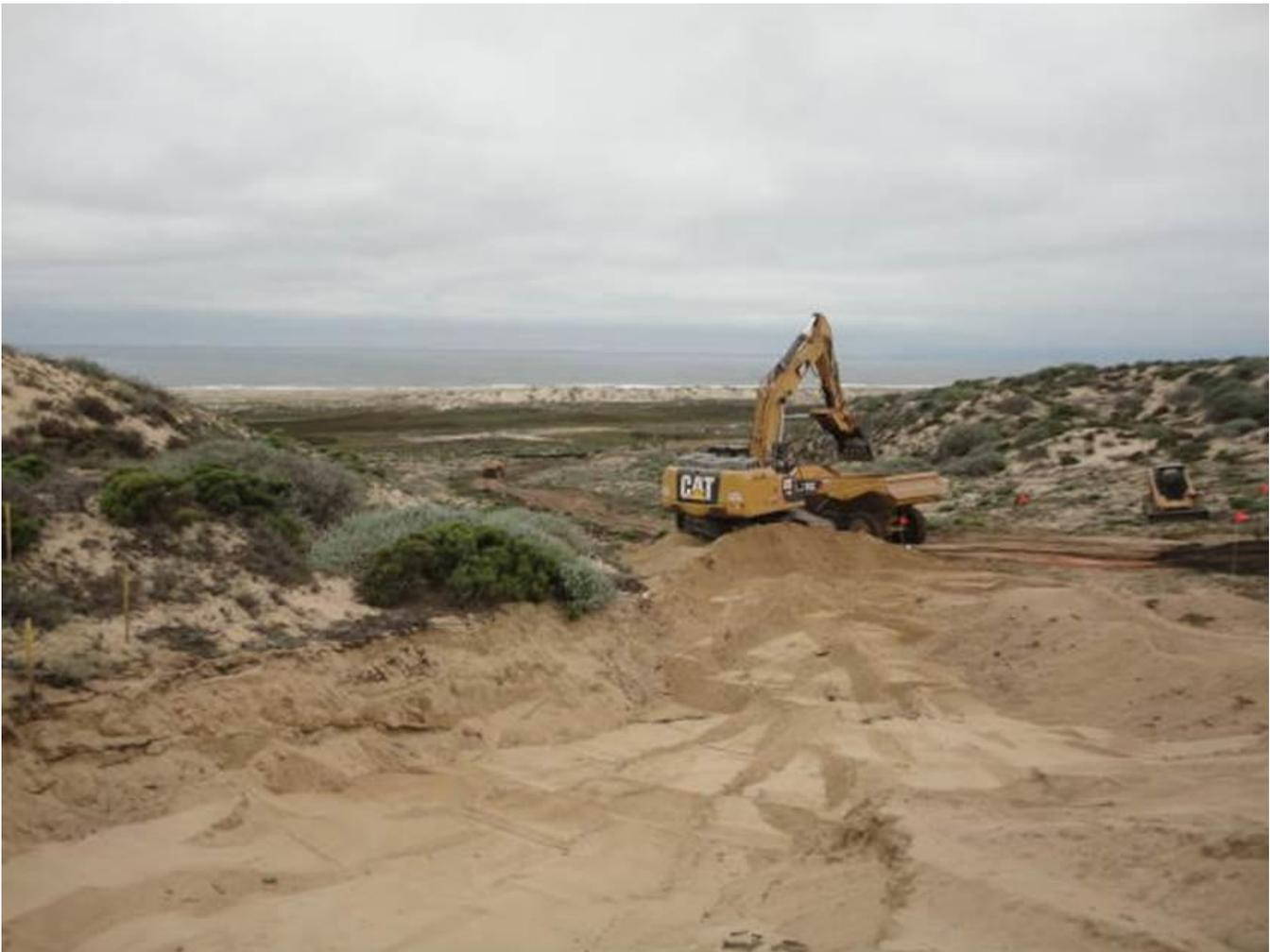
**The D12 PROS Pad Site: excavation of sump and diluent-affected material.**
