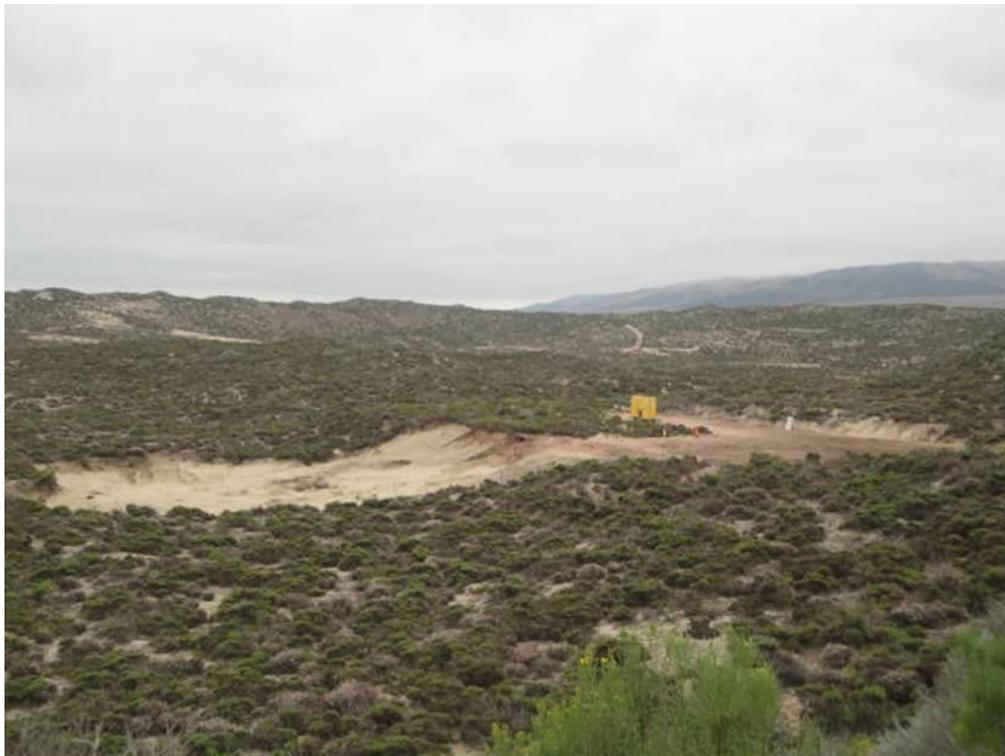
**The E1 PROs Pad Site: post-excitation: all sump material has been excavated from this site and will be backfilled after backfill approval from OEC and RWQCB.**
