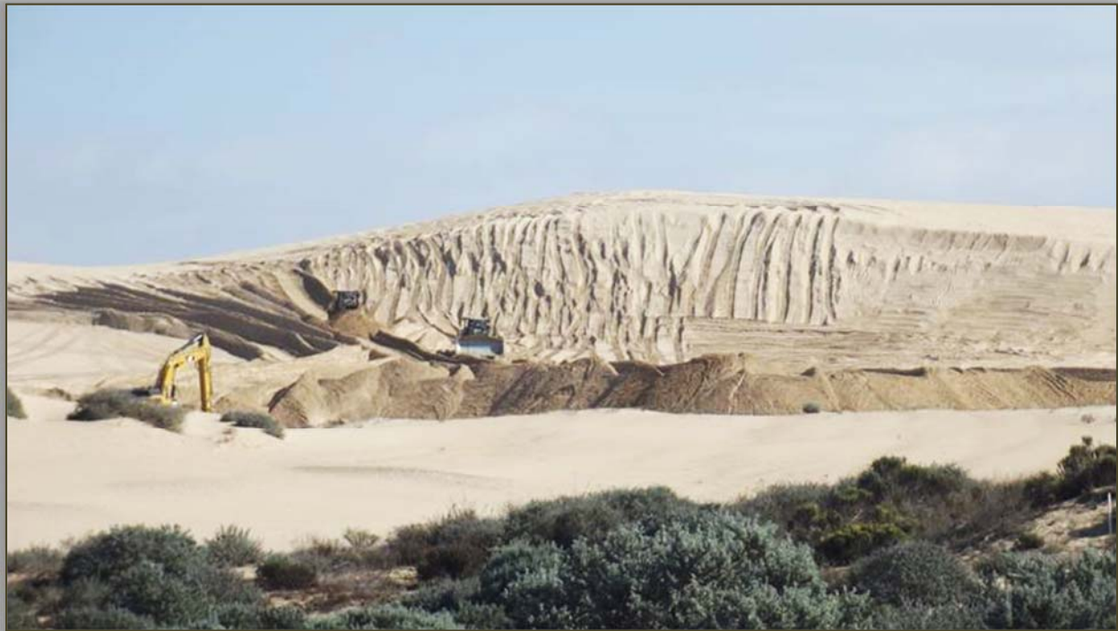
The Q4 Borrow Site: Chevron/Entact continues to use sand from this site for approved backfill material. Chevron requested permission and was authorized to temporarily regrade the area both within and outside the previously approved boundaries, to regrade the sand dunes within the approved borrow site boundaries and to reduce sand erosion outside of the area.
