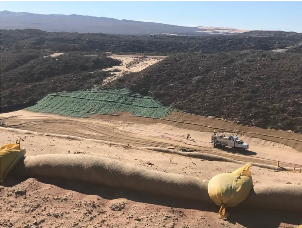
The M1 Valley: hydroseed being sprayed on jute-netting along steeper slopes.
