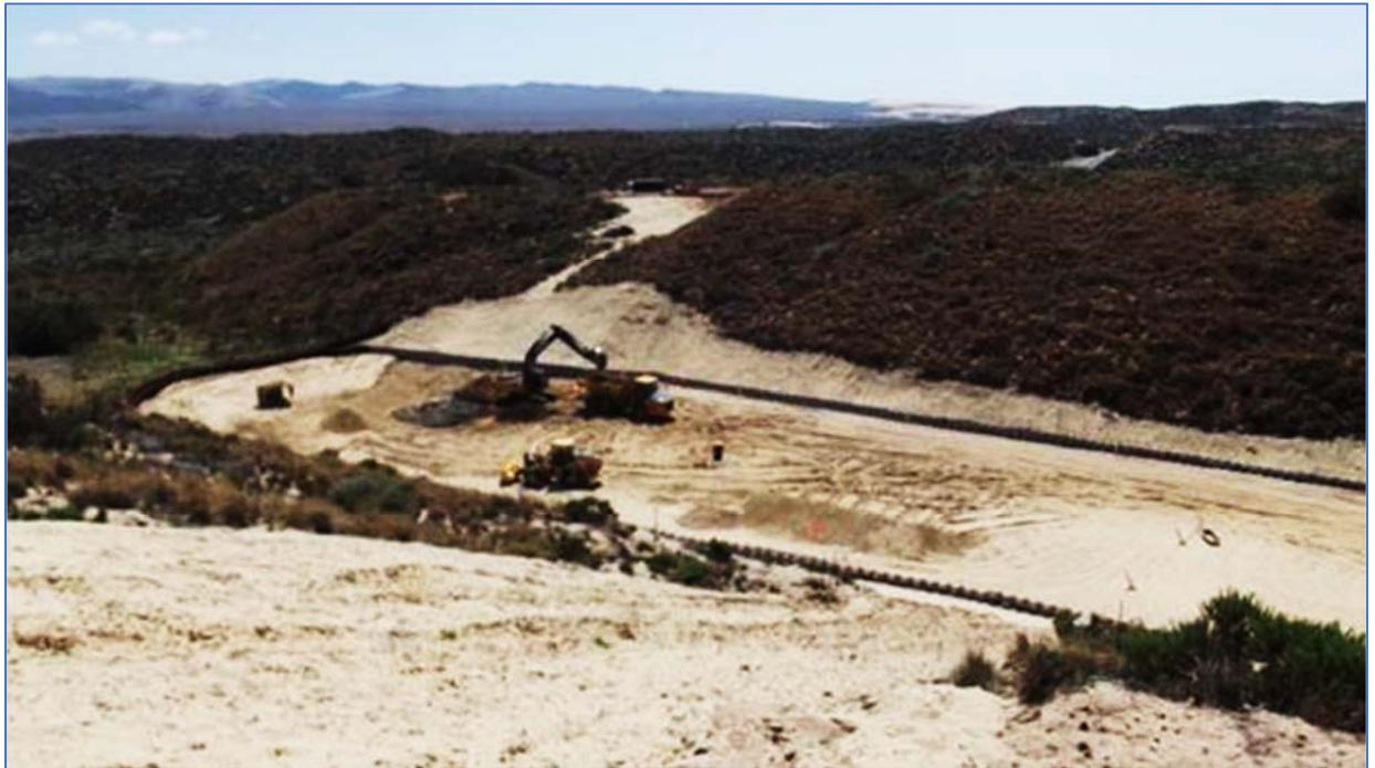
**The M1 Valley: excavation of diluent-affected material and temporary backfill to ensure that there is no potential for any wildlife exposure to contaminated soils and no standing water overnight.**
