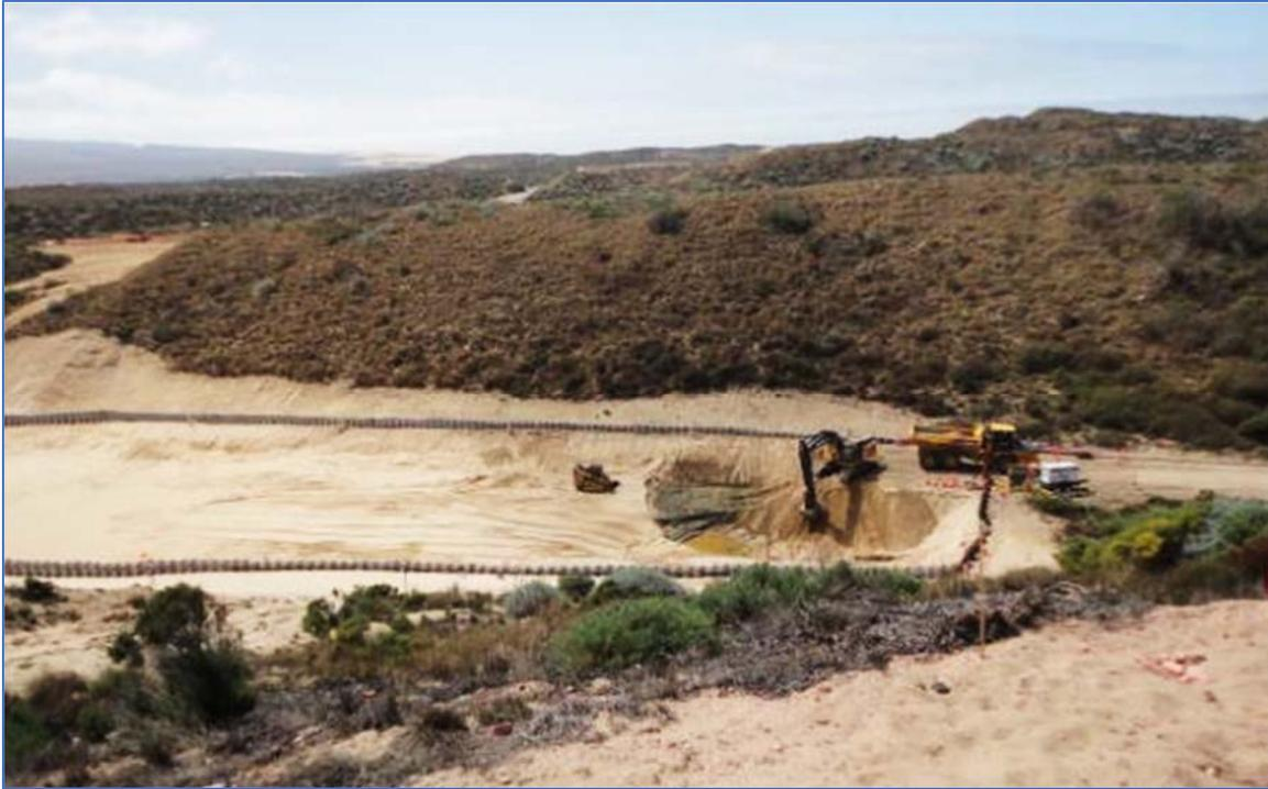
**The M1 Valley: excavation of diluent-affected material almost completed. Excavated areas are immediately covered with 6-10 inches of clean sand from the Q4 Borrow Site.**
