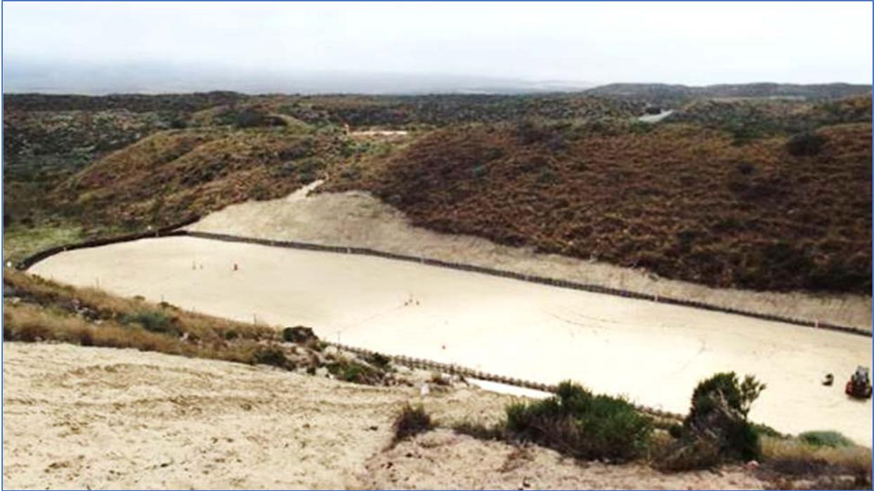
**The M1 Valley: both vinyl and steel sheetpile completely installed around the site.**
