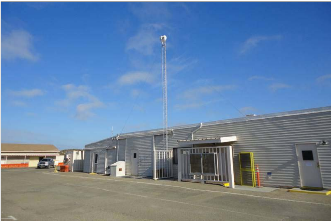
Newly installed antenna at the Guadalupe Field Station.
