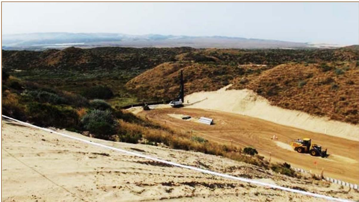
**The M1 Valley: sheetpile being installed around perimeter of site.**
