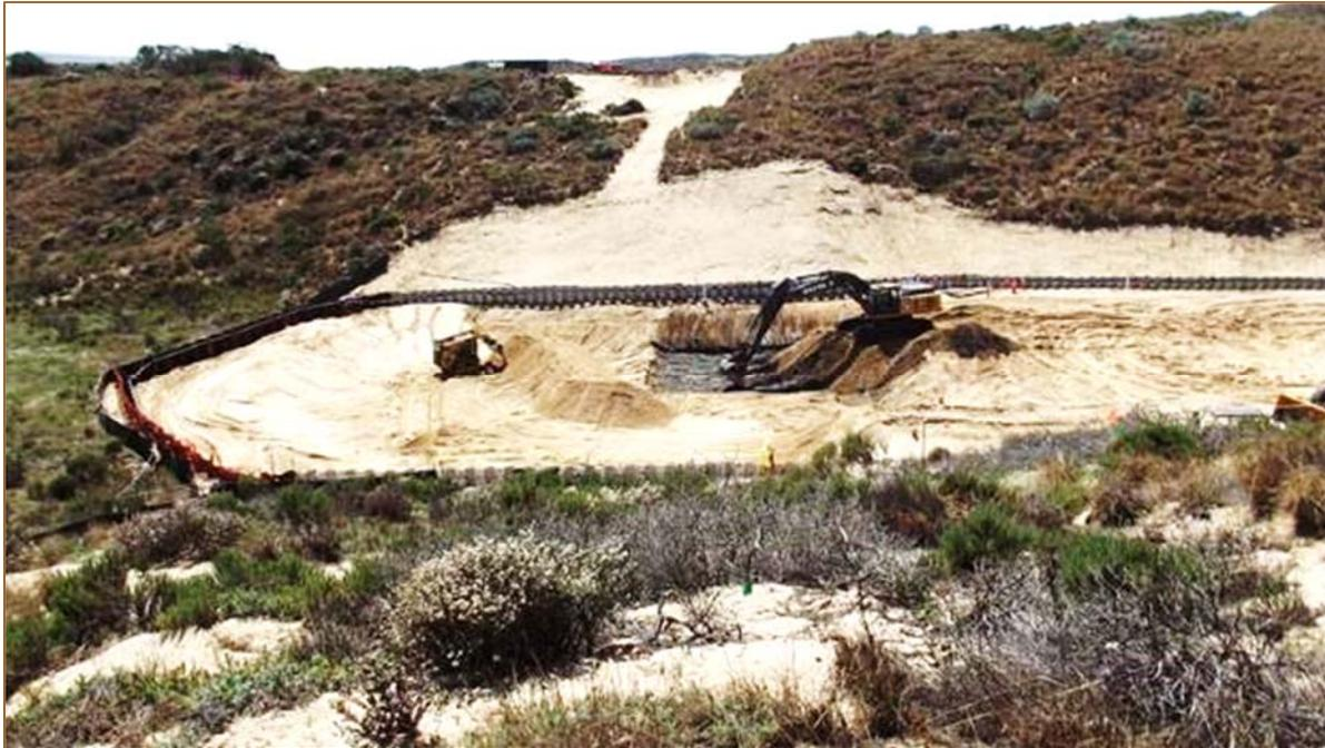
**The M1 Valley: excavation of diluent-affected material. Excavated areas are immediately backfilled with clean sand from the Q4 Borrow Site.**
