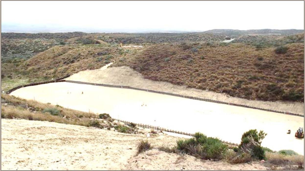
**The M1 Valley: both vinyl and steel sheetpile completely installed around site.**
