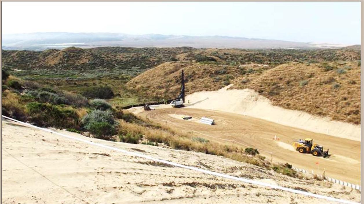
**The M1 Valley: sheetpile being installed around perimeter of site.**
