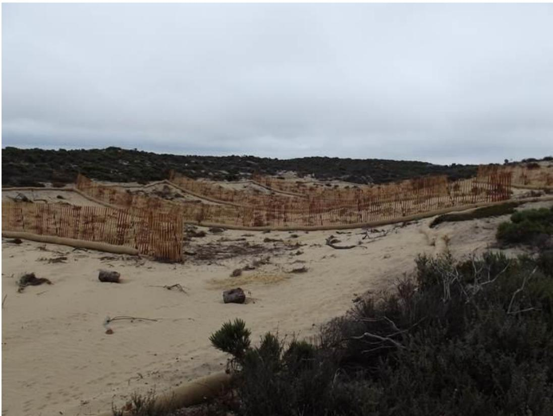
**The H5 Sump: post excavation activities and after sediment control measures have been installed.**
