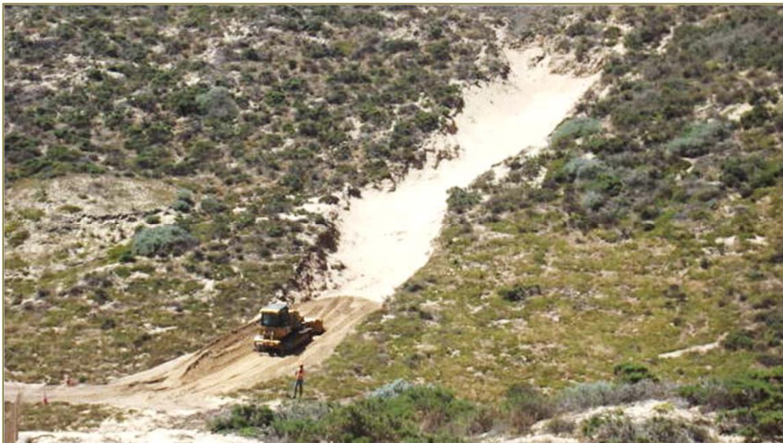
**G6 PROS Remediation Site: Same view as previous photo several weeks later. Chevron contractors have completed excavation and soil sampling, and are currently backfilling and regrading this site. After backfilling is complete, Entact will install sediment control measures including sand fence and vegetation (originally cut from the site) to help reduce wind and rain erosion from the steep slopes.**
