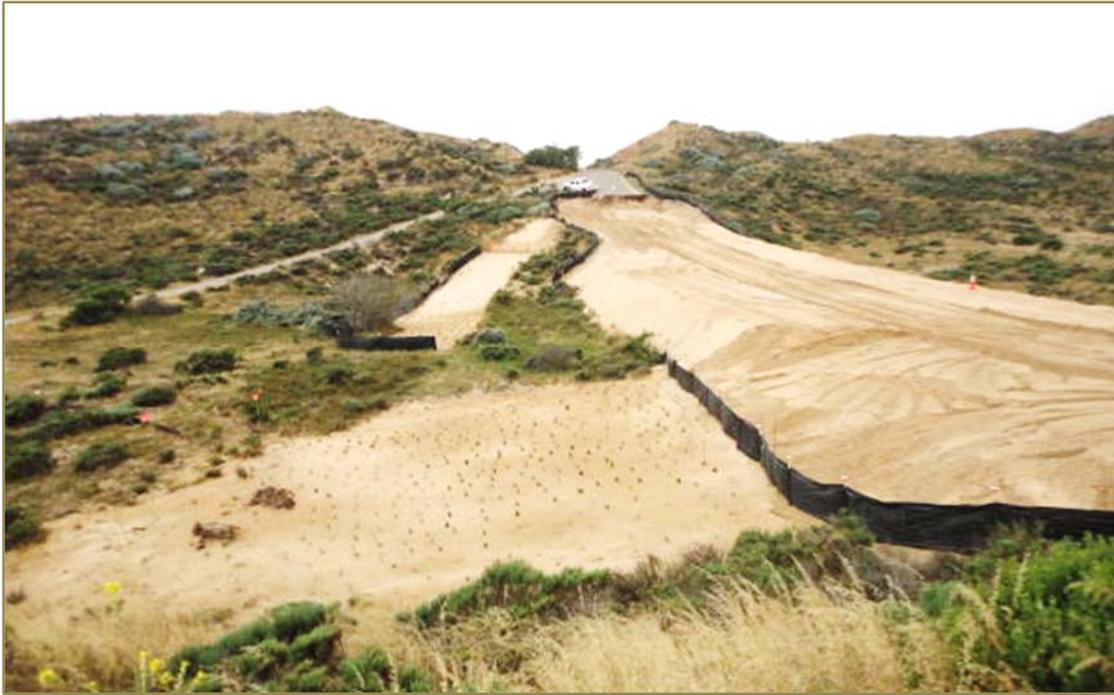
**L11 Road Work: the roadway was lowered and widened to permit haul trucks passage without further road degradation.**
