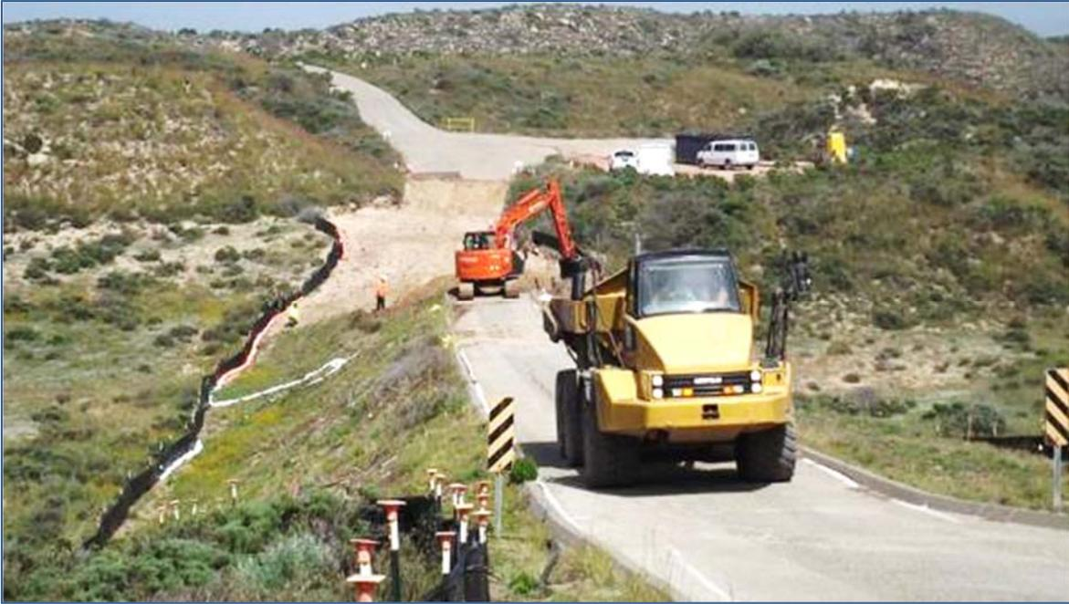
**L11 Road Work: Chevron contractors are currently lowering and widening this portion of the L11 Road to permit haul trucks passage without further road degradation.**
