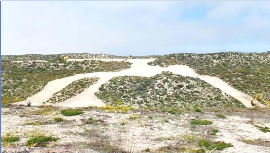
**G7 PROS Remediation Site: Chevron contractors continue to conduct PROS activities which include the excavation of contaminated material including sumps and diluent-affected materials extending off various Pad sites through-out the Field.**
